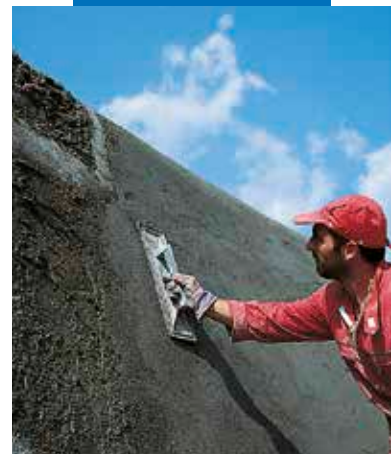
Finishing of Mapegrout T40
