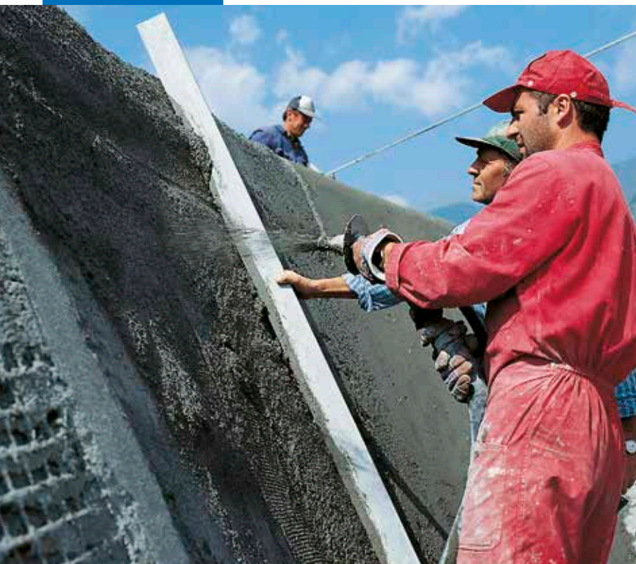
Spray application of Mapegrout T40
