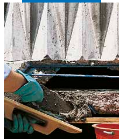
Repairing a balcony with Mapegrout T40
